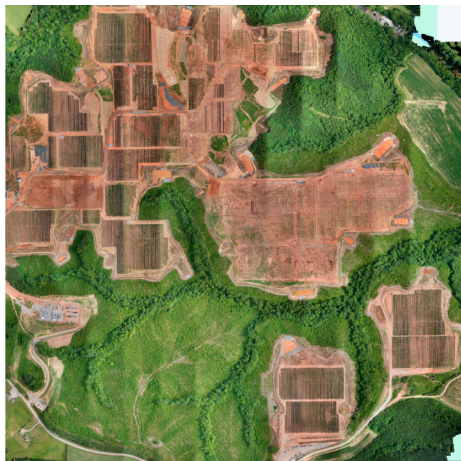
An aerial view of Capital Power's 35 MW Bear Branch Solar Project located near the Town of Walnut Cove. Construction is nearing completion with commercial operations anticipated in December.
