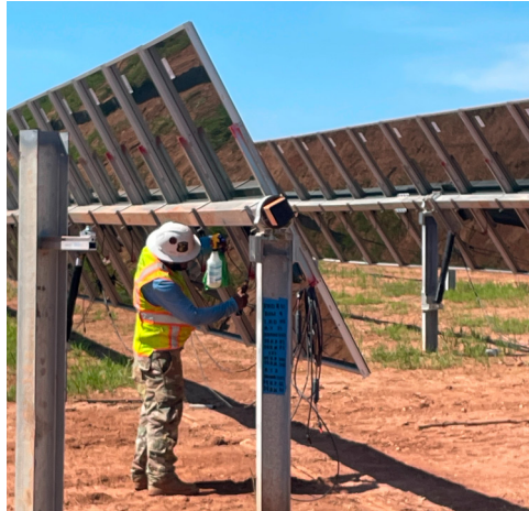
A worker installing one of Bear Branch Solar's 92,400 First Solar Series 6 Plus photovoltaic modules.
