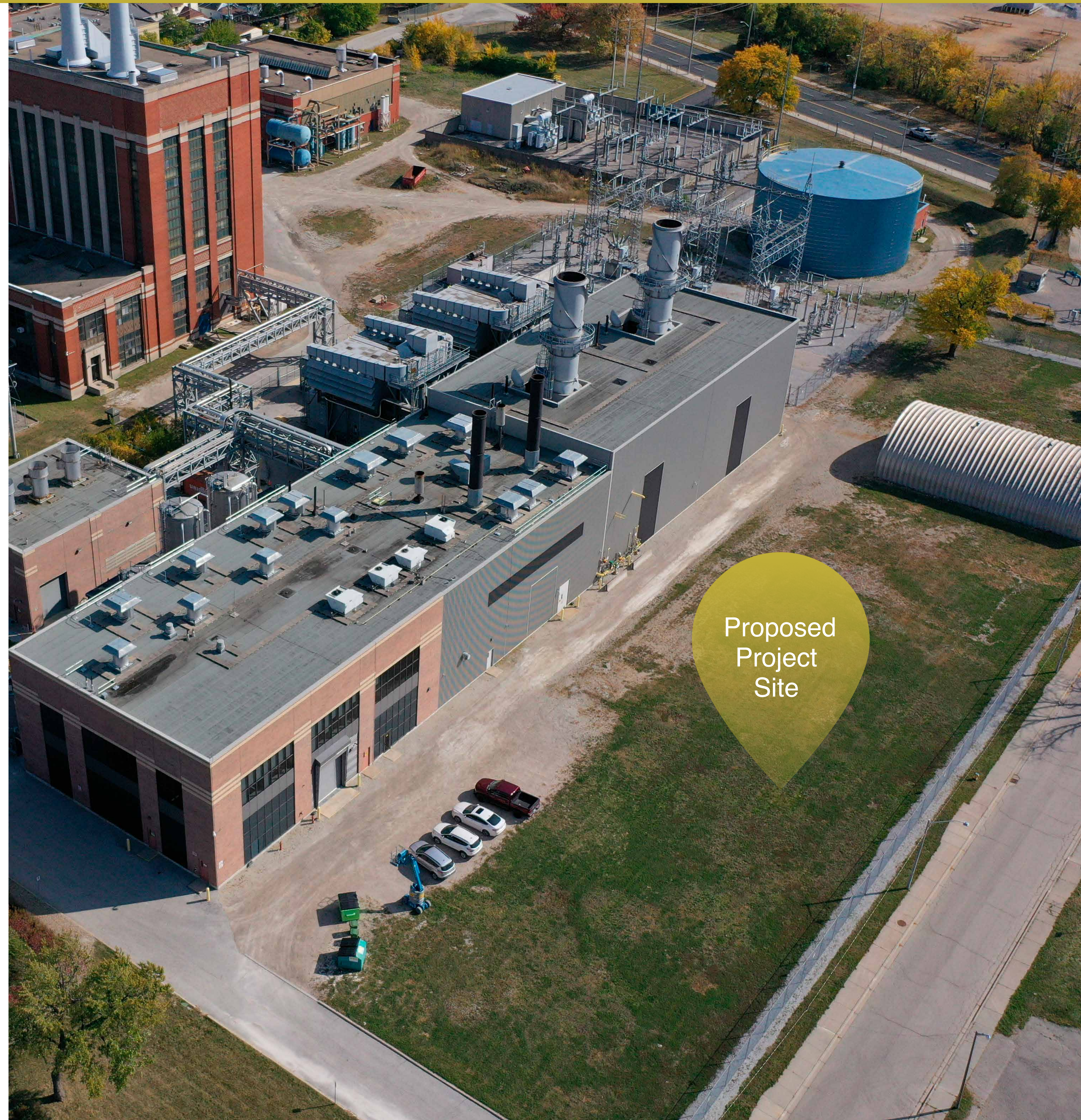
General project site
