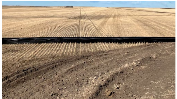
Erosion control measures along edge of a turbine pad under construction
