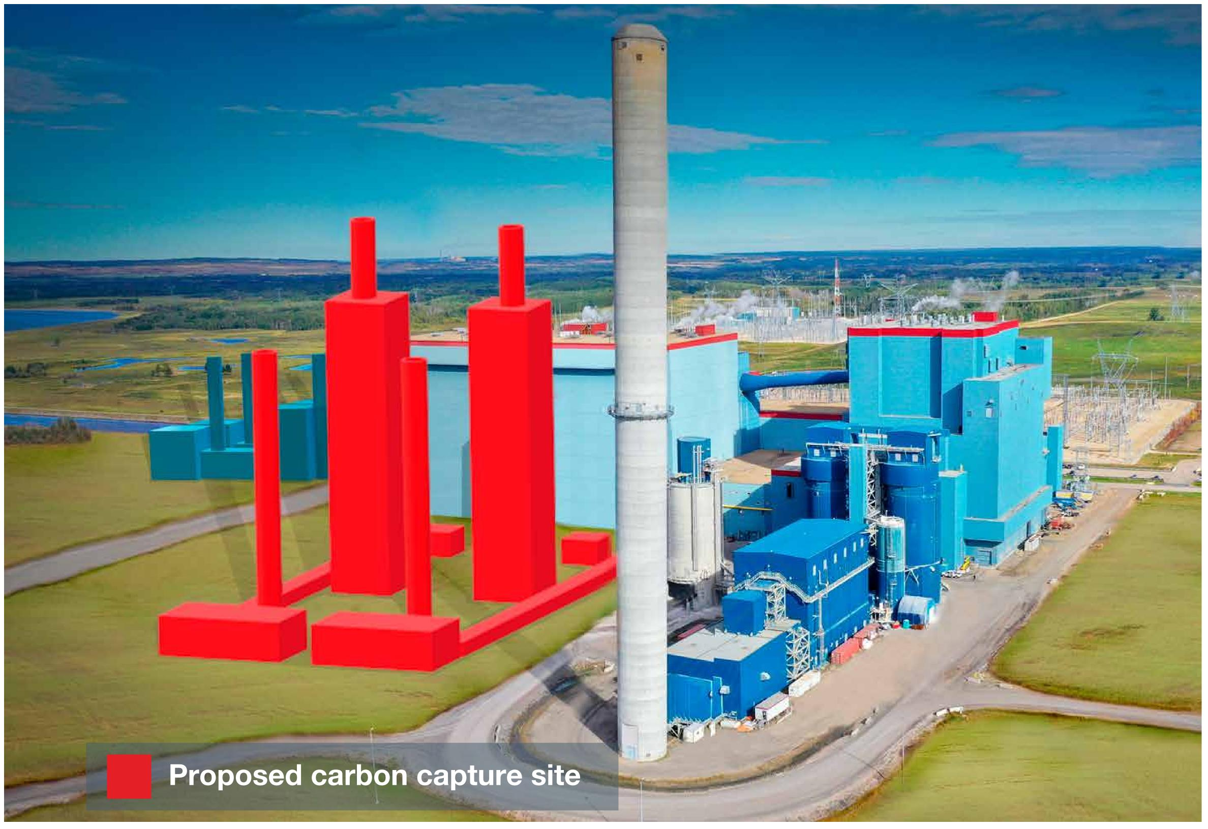
The square red towers are the carbon capture equipment's absorbers and are estimated to be ~280-ft high (pending final design) compared to the existing Genesee 3 stack that's ~456-ft high.
