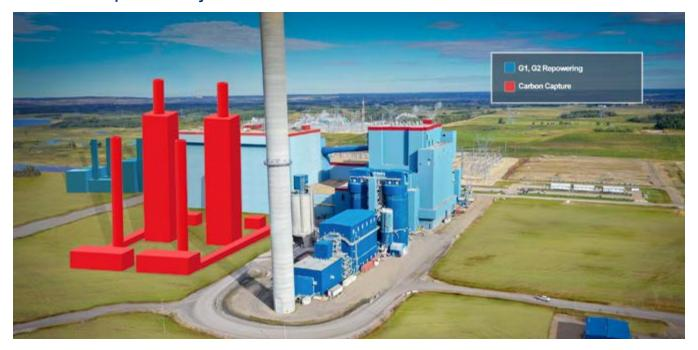
The equipment for the carbon capture project will be located on an approximately 10-acre brownfield site (previously developed land) on the south-side of Capital Power's existing Genesee Generating Station in an area where the coal and ash handling equipment are located. Some of this equipment will be retired and dismantled because it will no longer be needed following the transition from coal.
