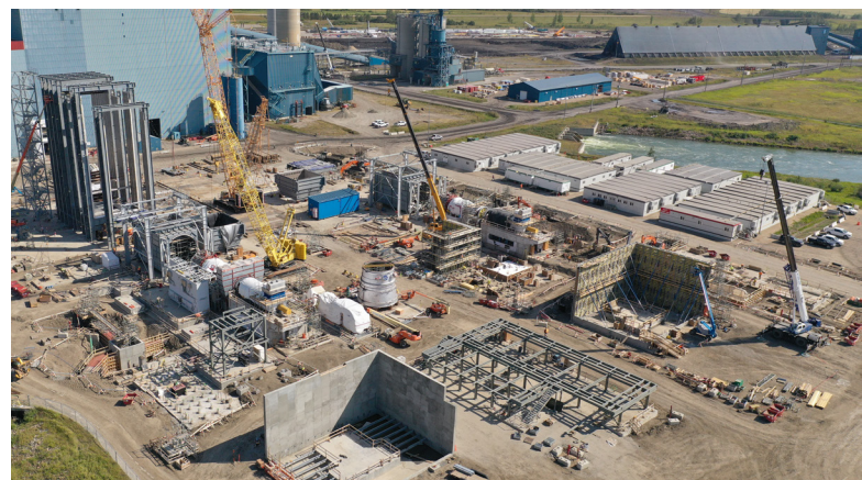
After a journey by ship, rail and road, the combustion turbine (CT) #1 and CT generator (CTG) #1, integral components of the Repowering Project, arrived at our Genesee Generating Station in February 2022.
