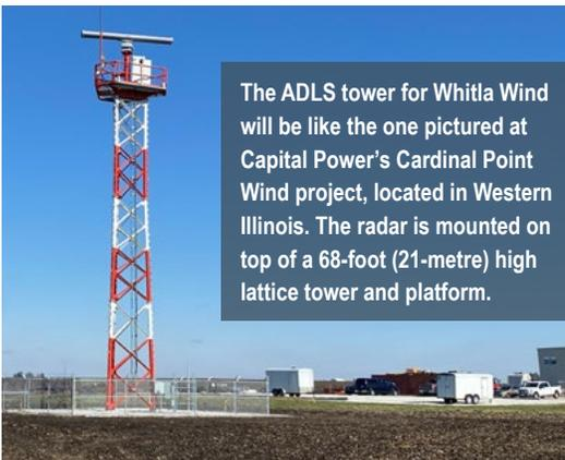
The ADLS tower for Whitla Wind will be like the one pictured at Capital Power's Cardinal Point Wind project, located in Western Illinois. The radar is mounted on top of a 68-foot (21-metre) high lattice tower and platform.
