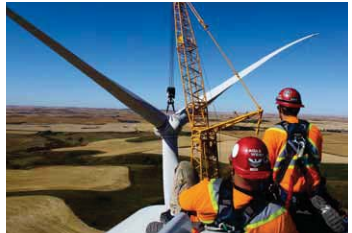
Skilled operators delicately position equipment into place.
