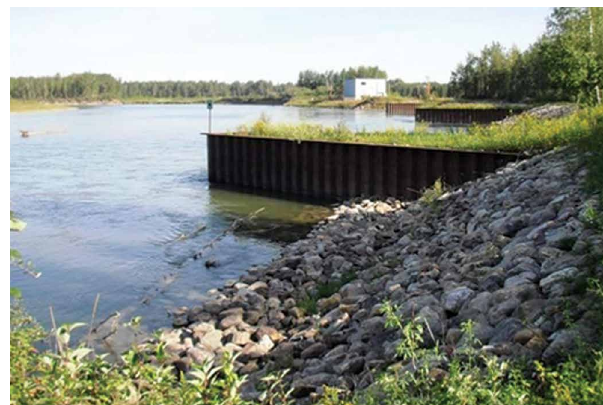
Photos of the intake and outfall structures for GGS. No changes are proposed to this infrastructure for the Project.
