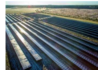
Beaufort Solar (100% of 15 MW capacity contracted)
