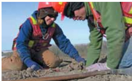
Julia Wachowski and Eckehart Marenholtz installing soil temperature sensors.
