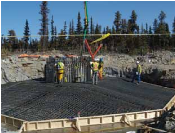
A typical concrete pouring of wind turbine foundation.
