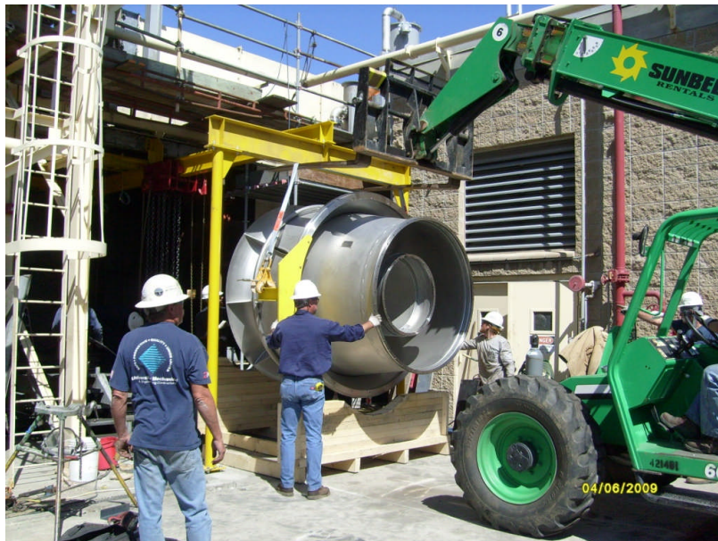
Diffuser installation
