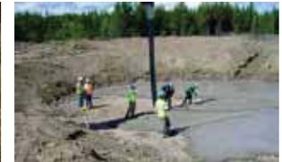
**Mud mat installation (to provide a level surface for the rebar).**
