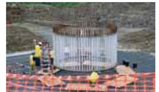
**Anchor bolt cage installation.**
