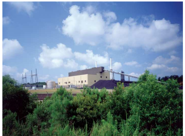
The electrical output from the Southport facility is sold under a Power Purchase Agreement to Progress Energy.
