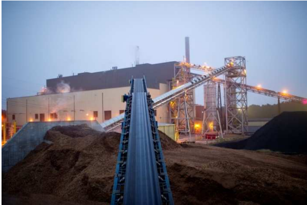
Southport uses a mixture of wood residuals, tire-derived fuel and coal to create electricity.
